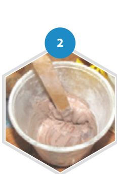
Mix According To The Specified Ratio
