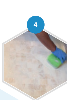
Lightly Clean Off Excess Grout With Wet Sponge
