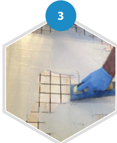
Apply Grout With Float
