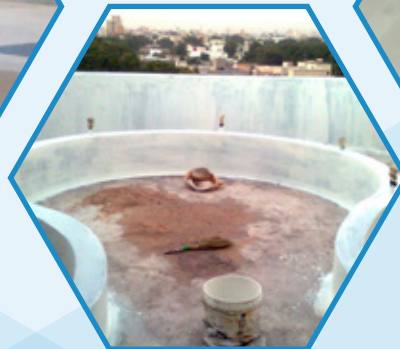
Terrace Garden Waterproofing
